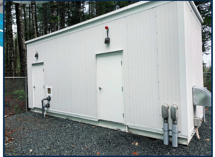
Figure 1: Exterior after installation
